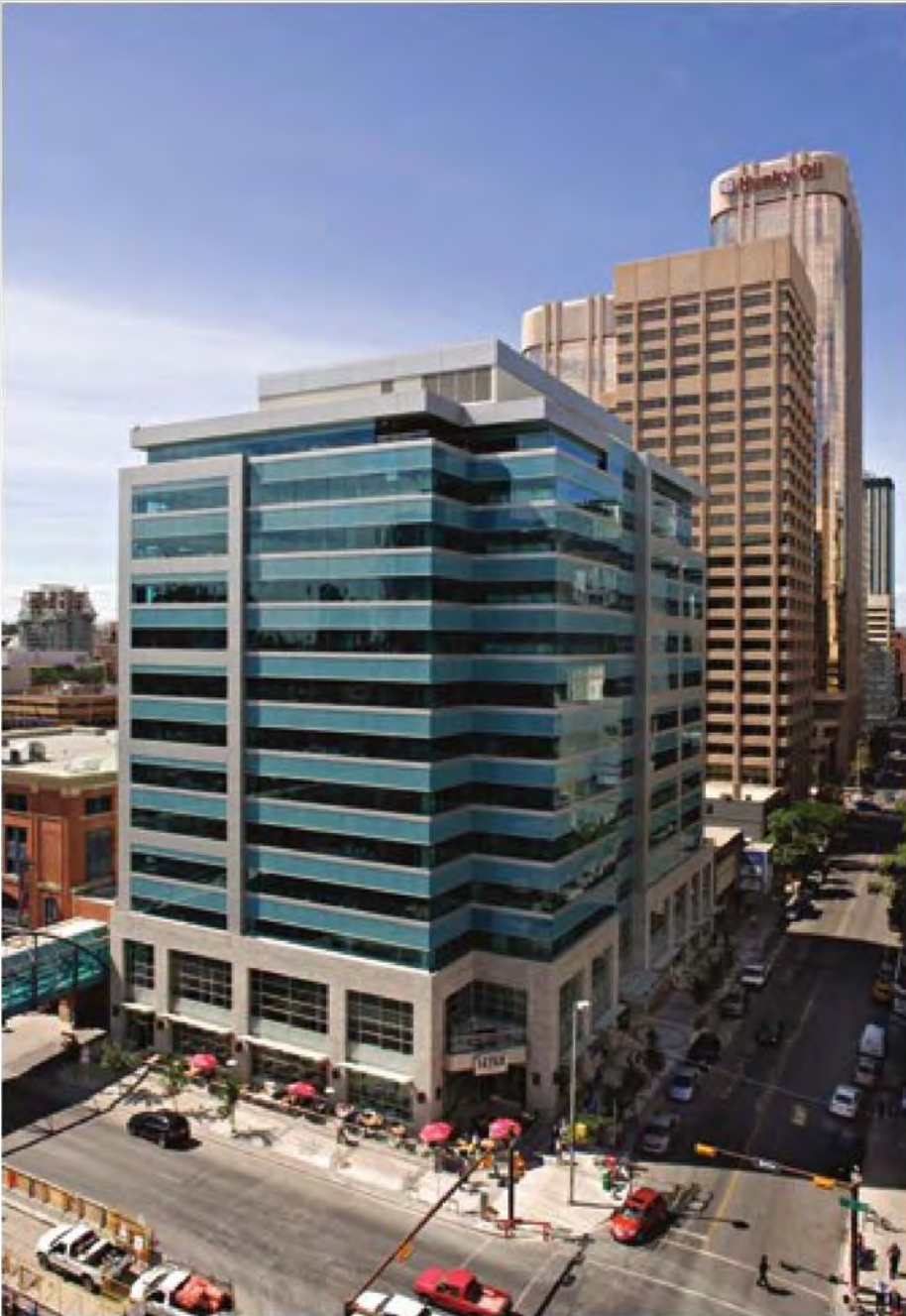
OPUS 8 office tower, developed by OPUS Corp (photos courtesy of OPUS)
